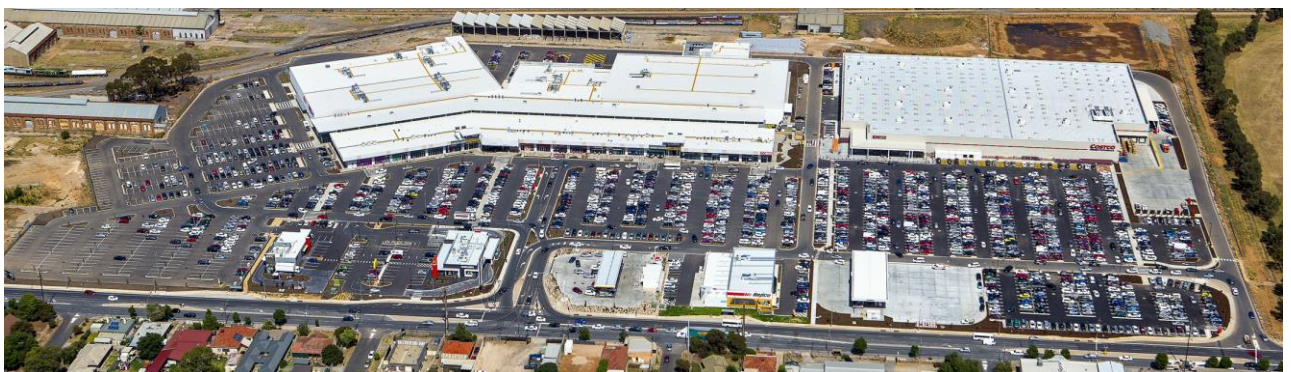
Churchill Centre North
