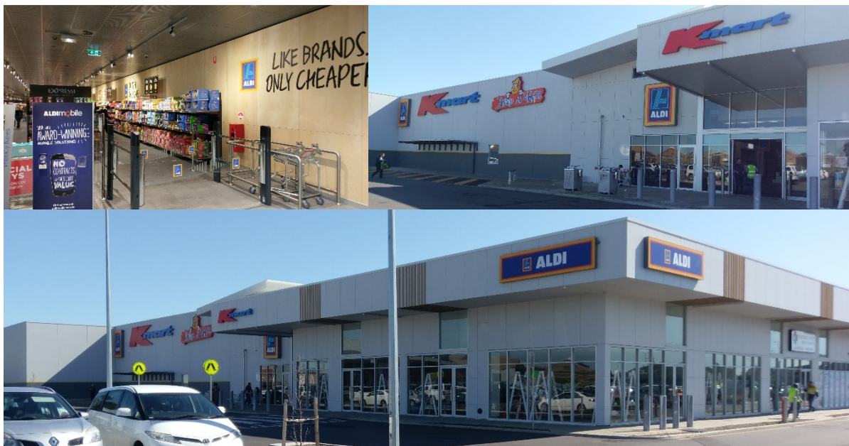
Churchill Centre North Aldi extension
