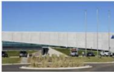
Perimeter Technology Oklahoma City 22,000 SF
