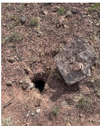
Photo-3. DH1005 historic drillhole at the Red Hill project, before the improvement.
