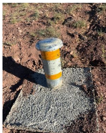
Photo-4. DH1005 historic drillhole at the Red Hill project, after the improvement.
