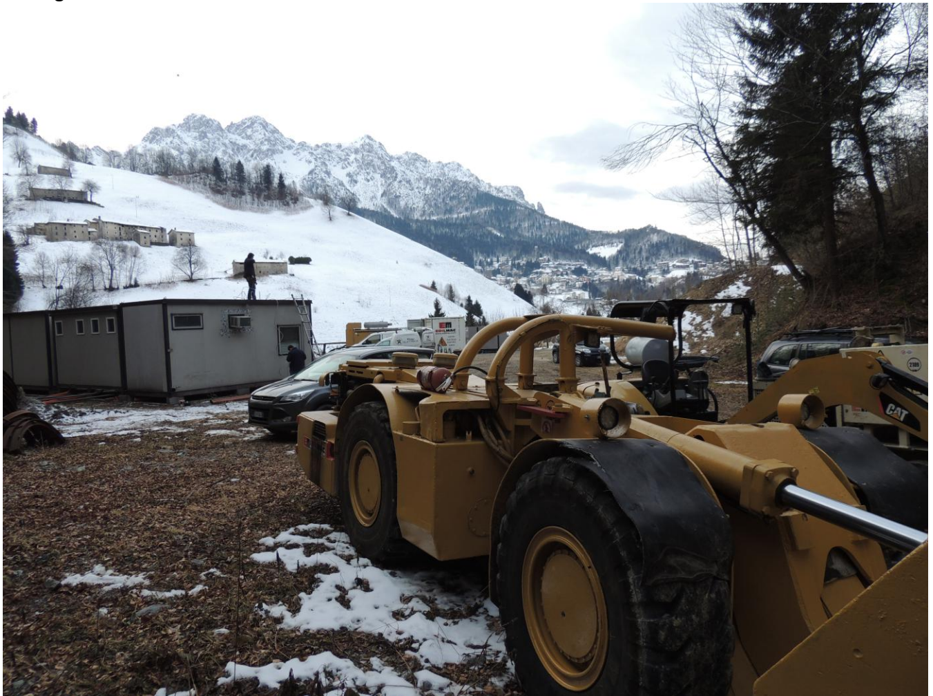
Site office and Laydown area for commencement of works
