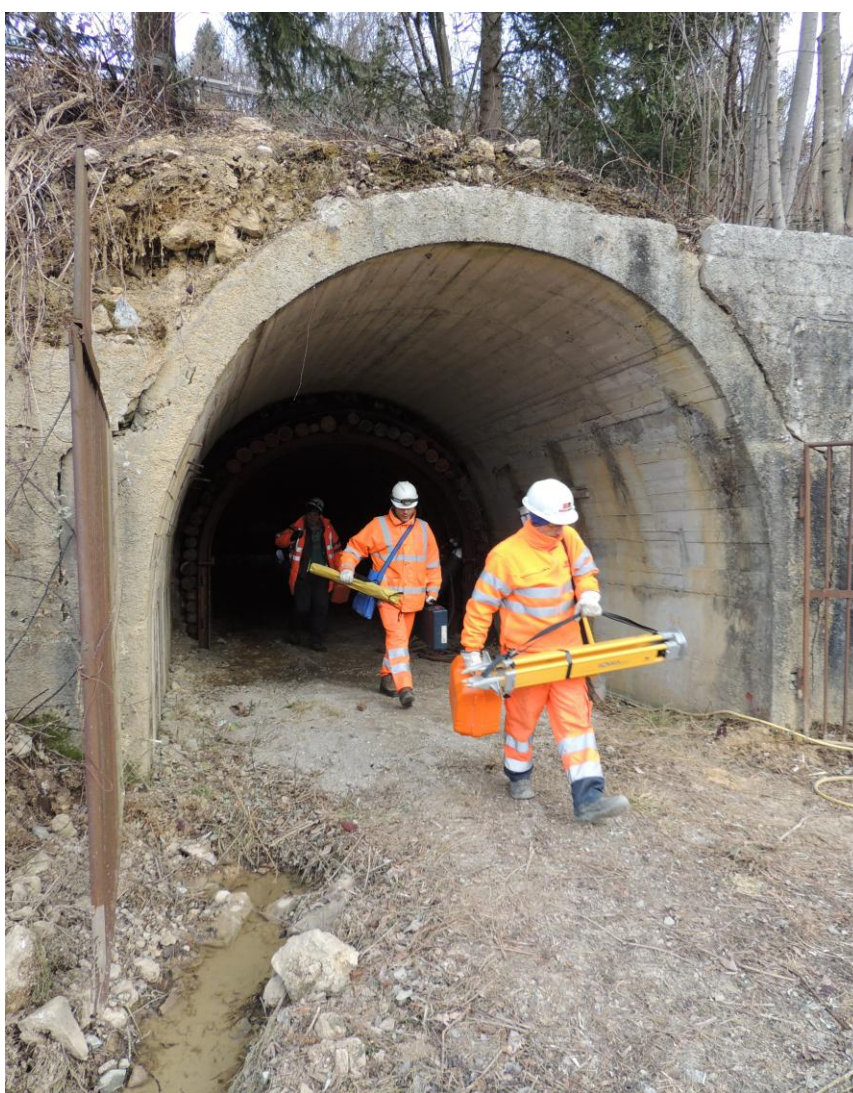
Underground Surveyors commencing works in the Access Tunnel
