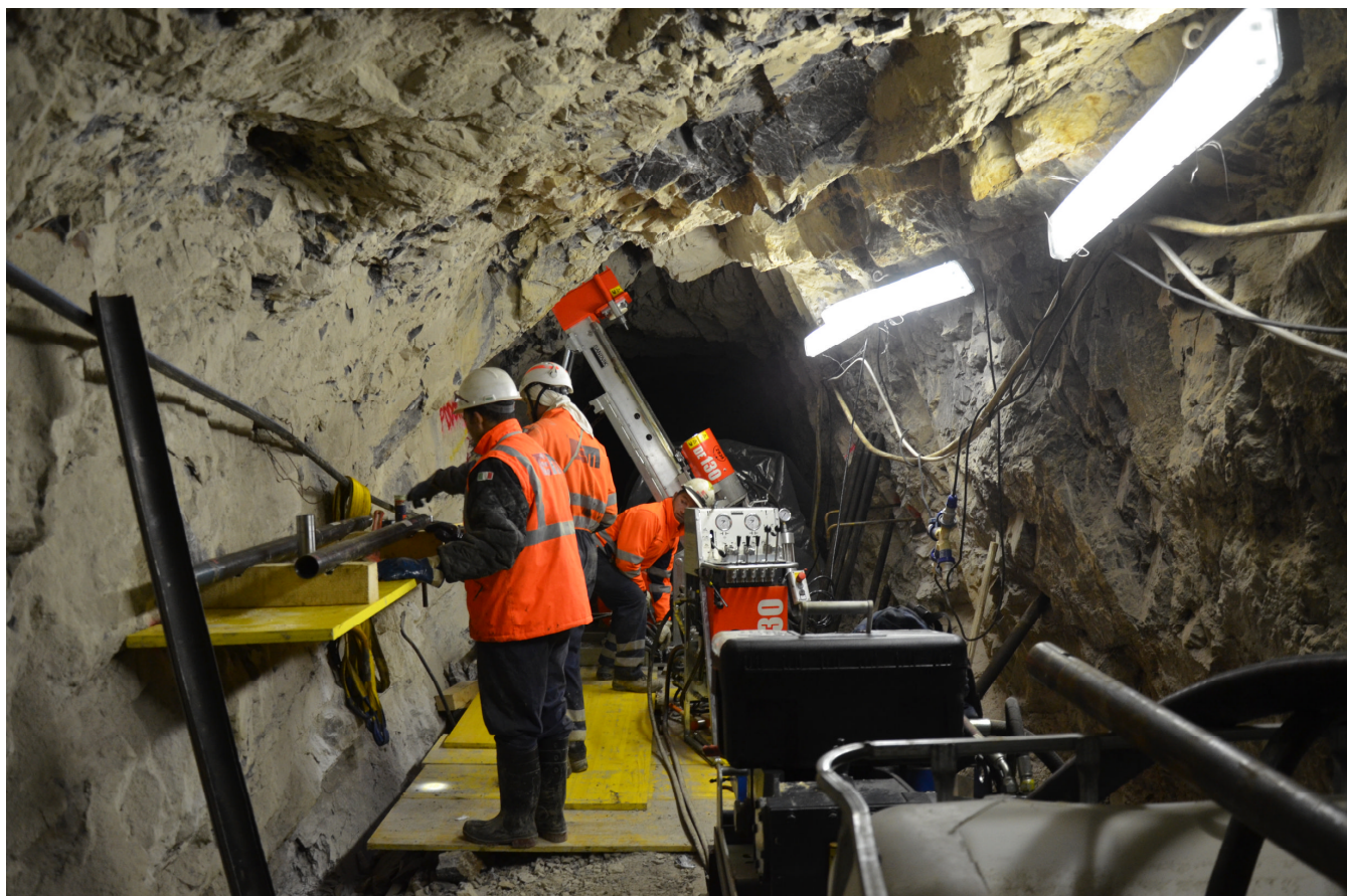
Figure 3: Sandvik rig being prepared for drilling on the 940RL level beneath the Colonna Zorzone zinc deposit
