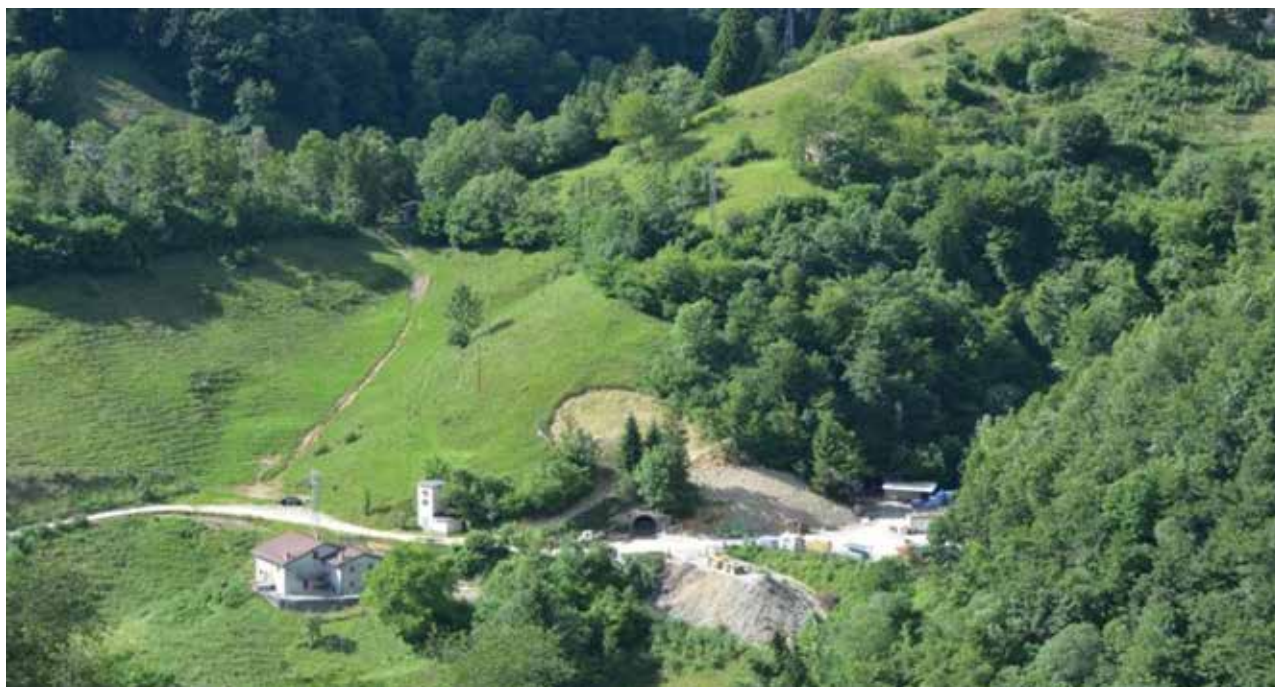
Figure 3 – Gorno Zinc Project, showing recent development and rehabilitation at the Ca Pasi entrance to underground workings
