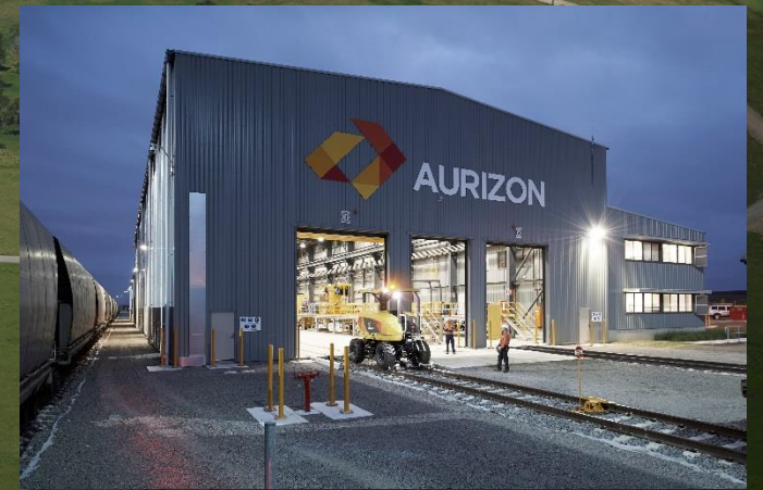
Hexham Train Support Facility, New South Wales
