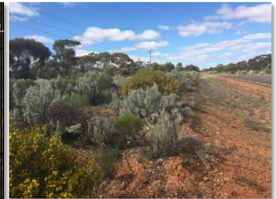
Mains Power (L) and Bulung Road (R)
