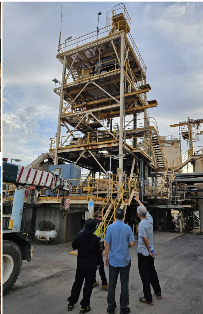
Figure 3: Sundry representatives inspecting refurbishment at Paulsens
