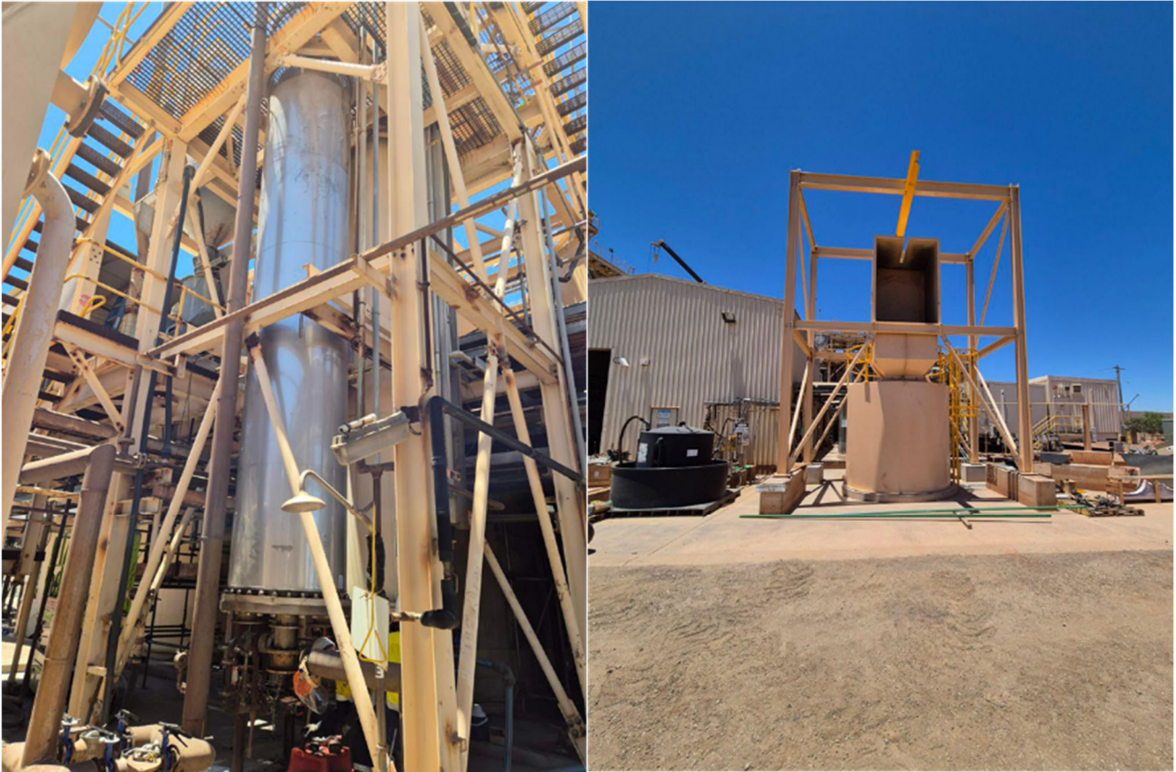
Figure 5: The newly constructed and installed cyanide mixing facility and the new elution column installed in position.
