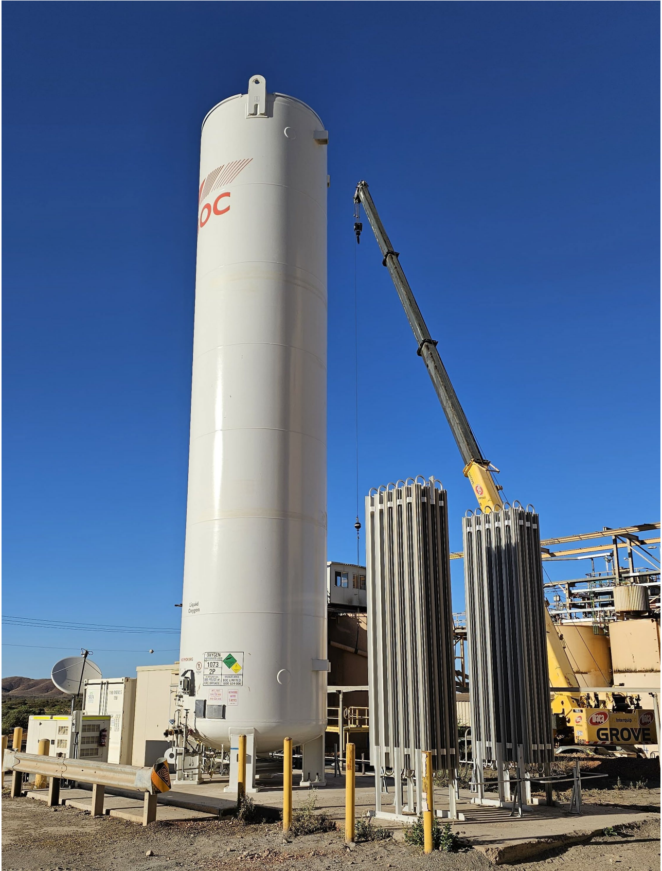
Figure 5: Showing the newly installed oxygen storage tank.
