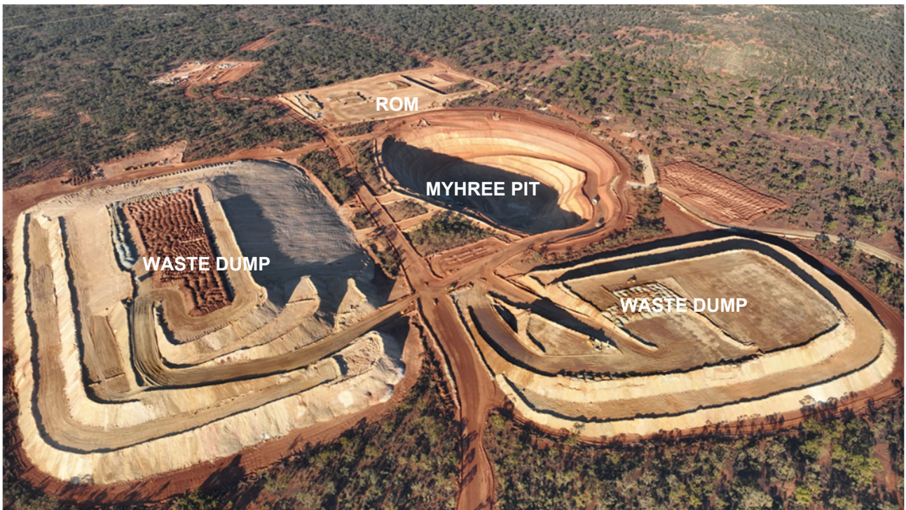
Figure 4: Myhree open pit (looking south) has been mined to 310mRL with rehabilitation underway on the eastern waste dump.
