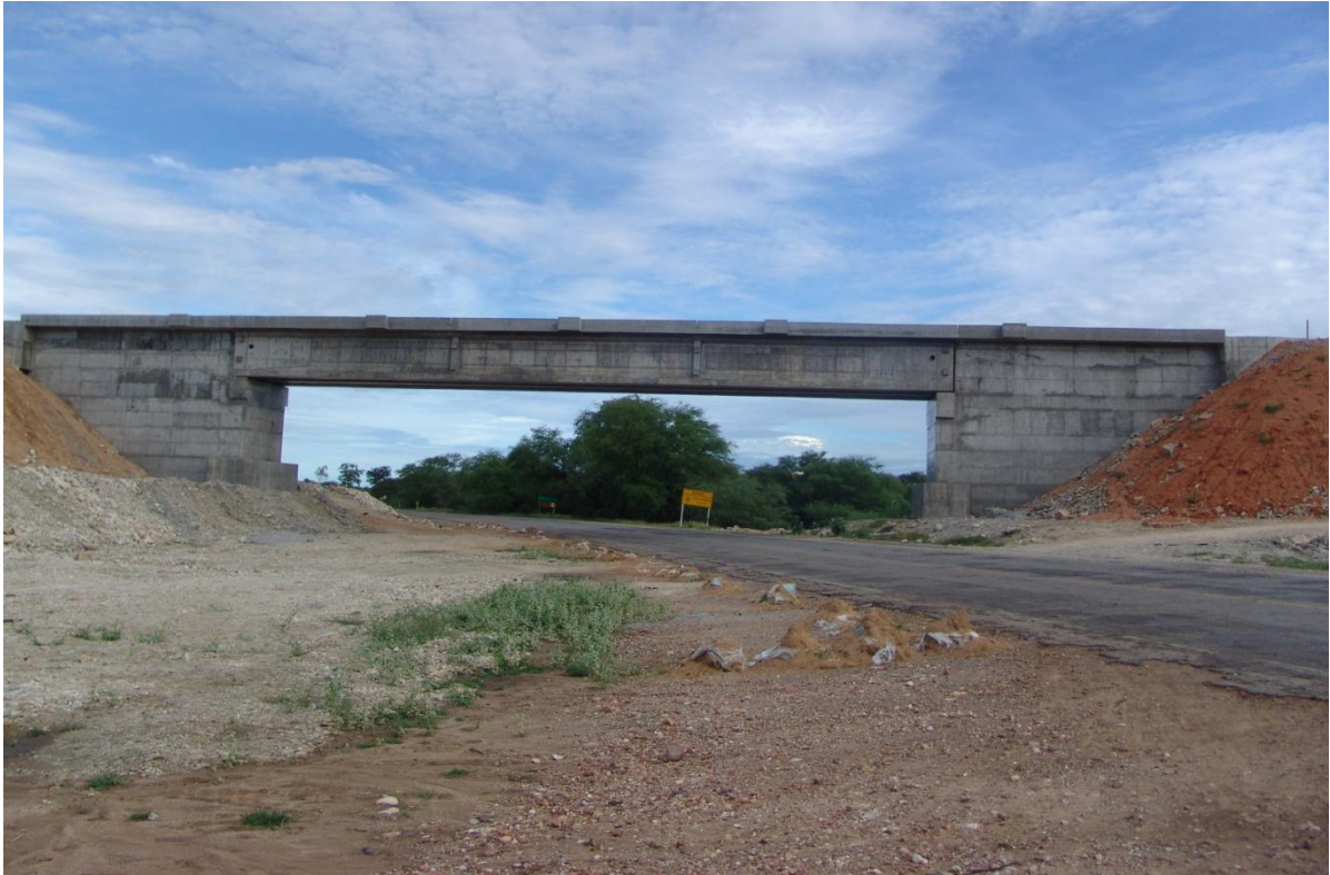
Photo: Overpass constructed for FIOL rail line between Brumado township and Cabral's Sincorá Area
