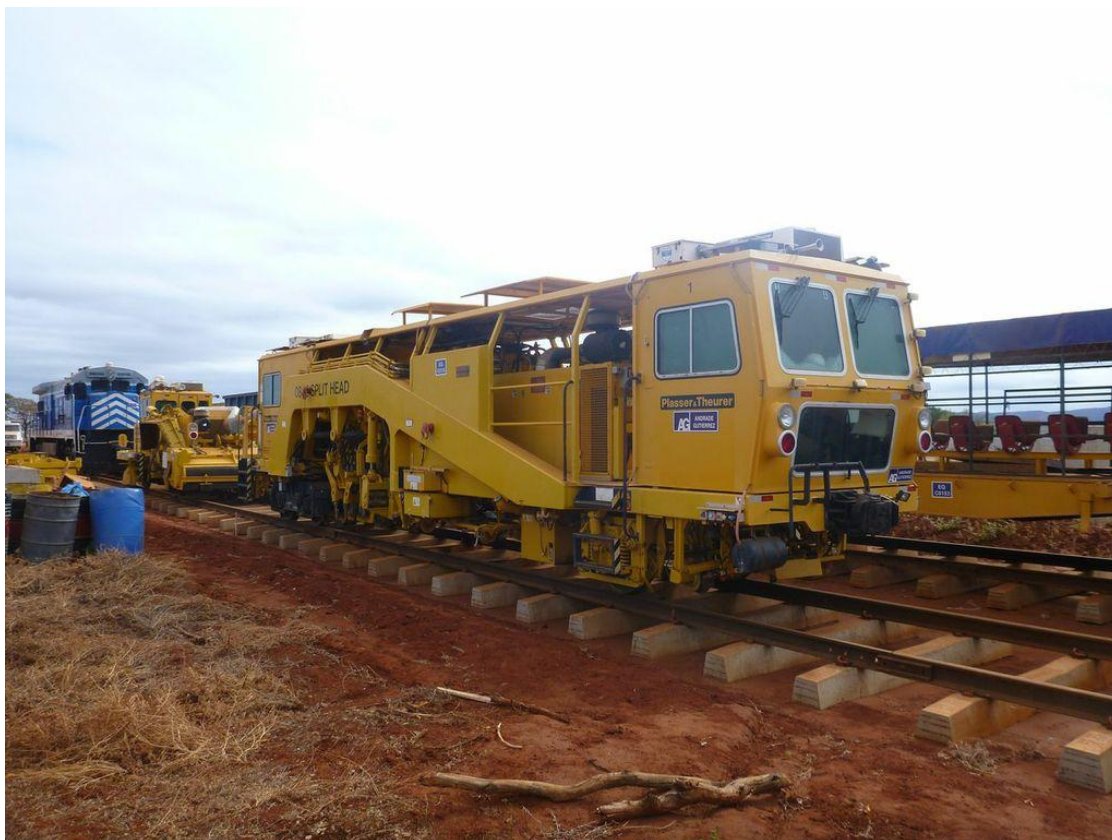
Current construction progress at FIOL Rail Line Lot 4, close to Cabral's tenements.
