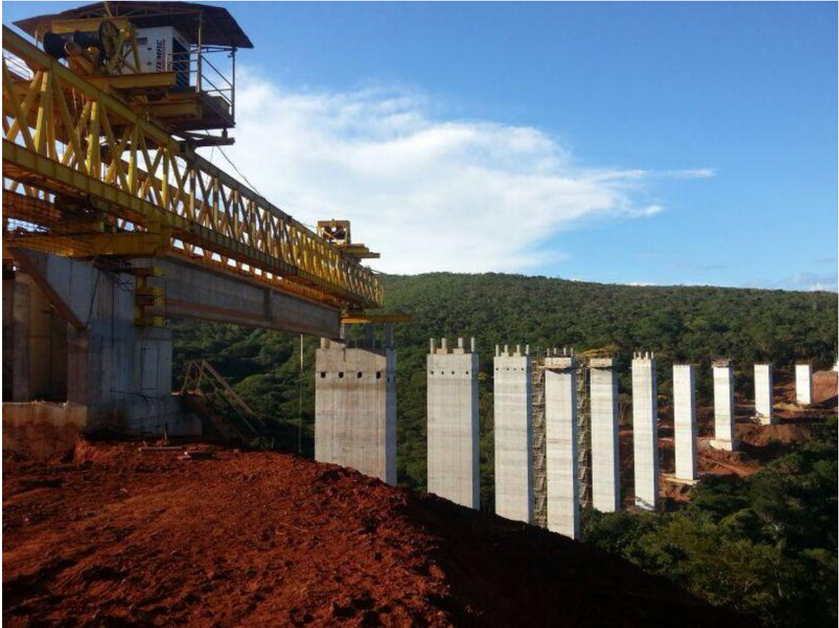
Photo: Progress in the construction of FIOL Rail Line.
