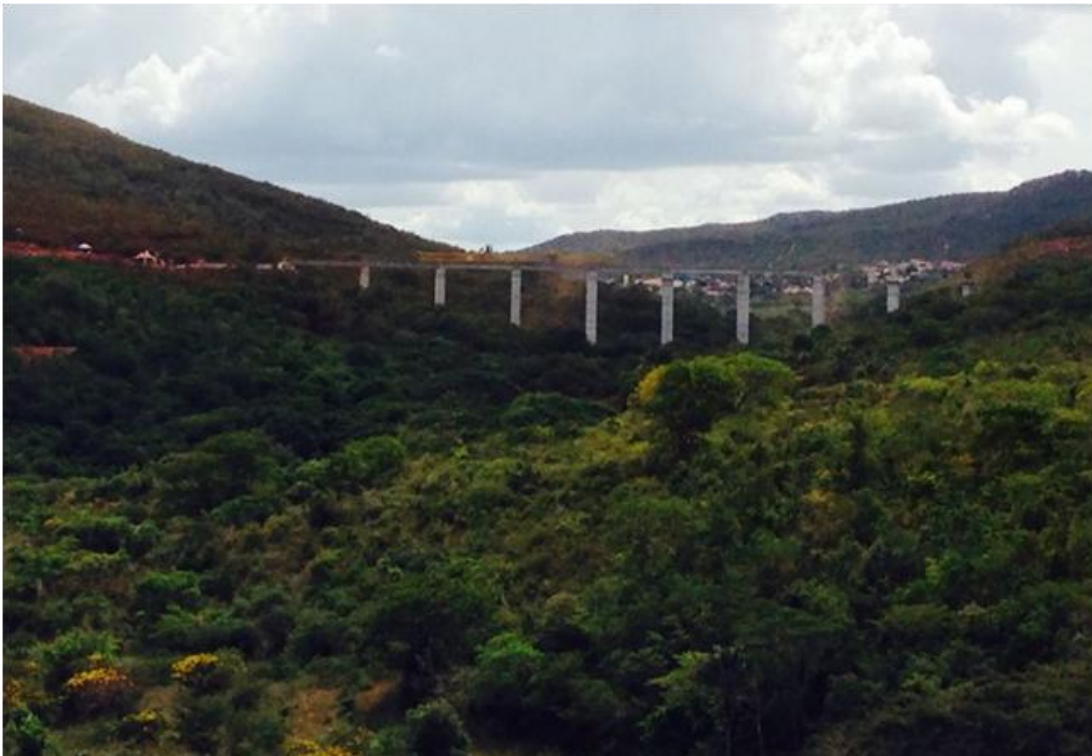
Photo: Progress in the construction of FIOL Rail Line.
