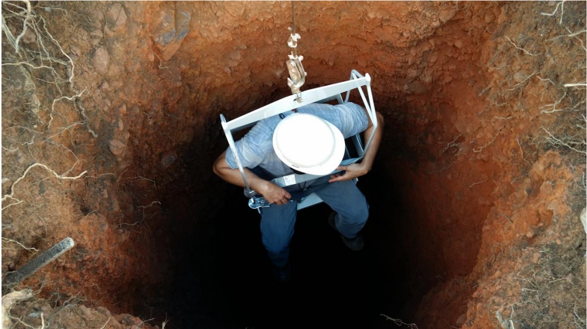
Photo: Cabral's Head of Exploration, Paulo Ribeiro, descending down QXD Pit 1 to its completed depth of 7.90m.
