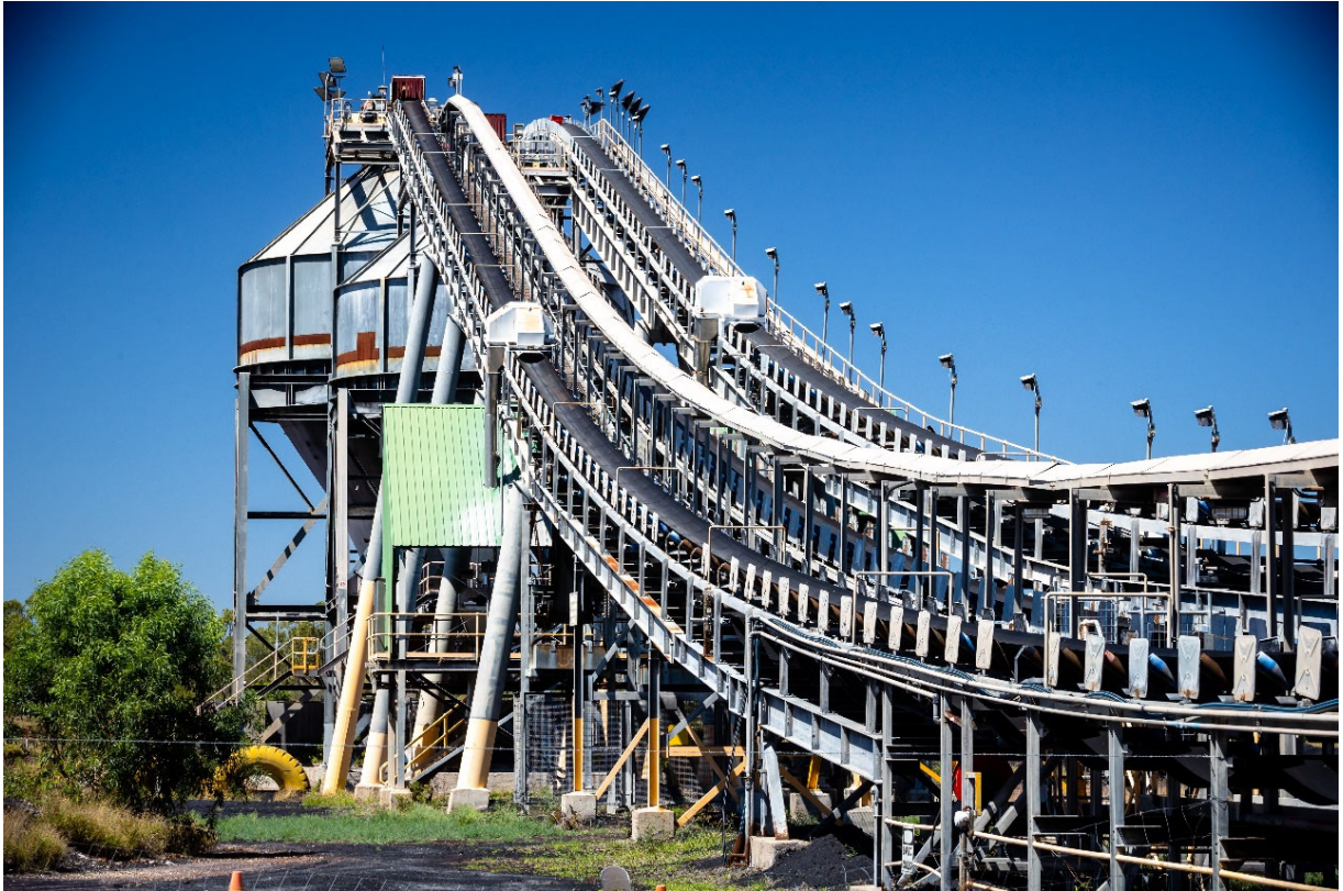
The Burton Infrastructure Complex. Source: Bowen Coking Coal.
