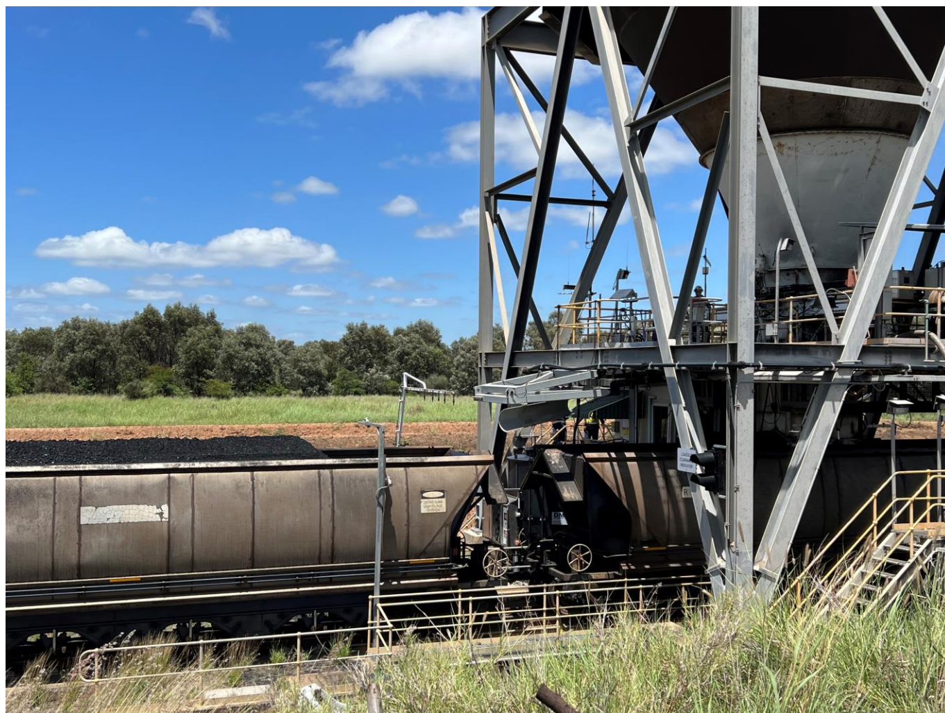
Figure 4: First coal being loaded through the Mallowa Train Loadout Facility, part of the Lenton Joint Venture.
