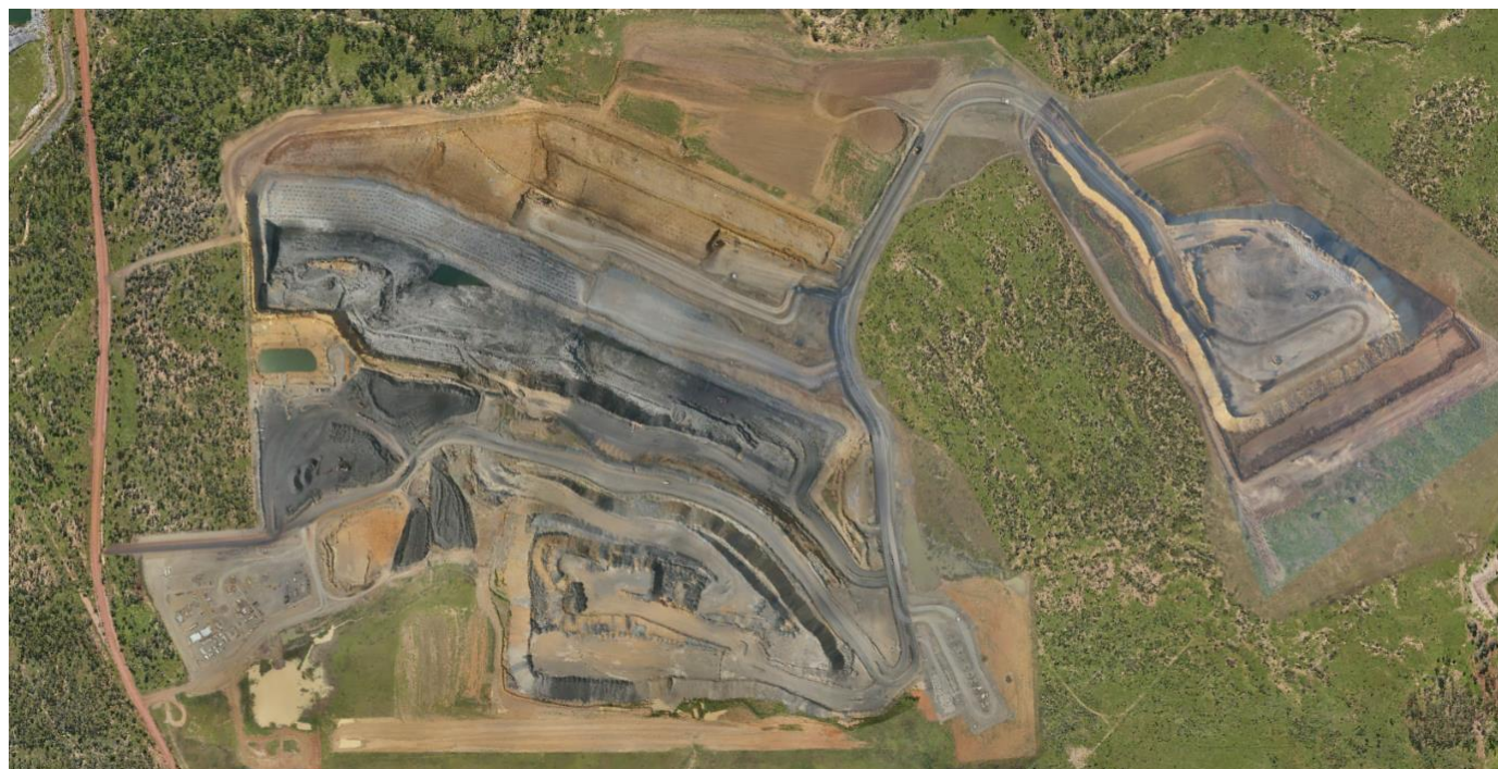
Figure 2: Broadmeadow East Pit, aerial view March 2023.
