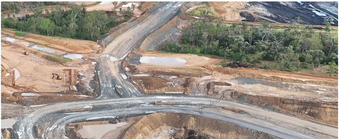
Figure 2: Teviot Creek Crossing Construction (looking North)
