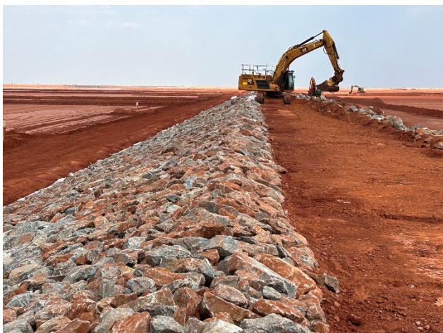
Image 3: Rock embankment construction
