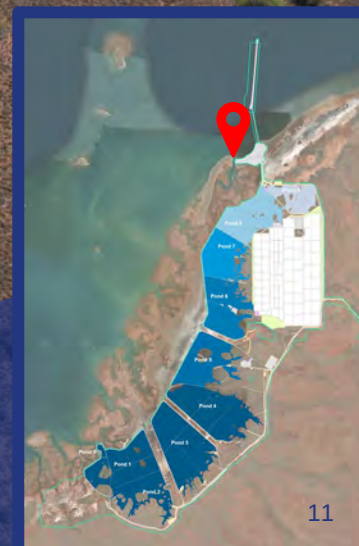
Construction of the secondary seawater intake
