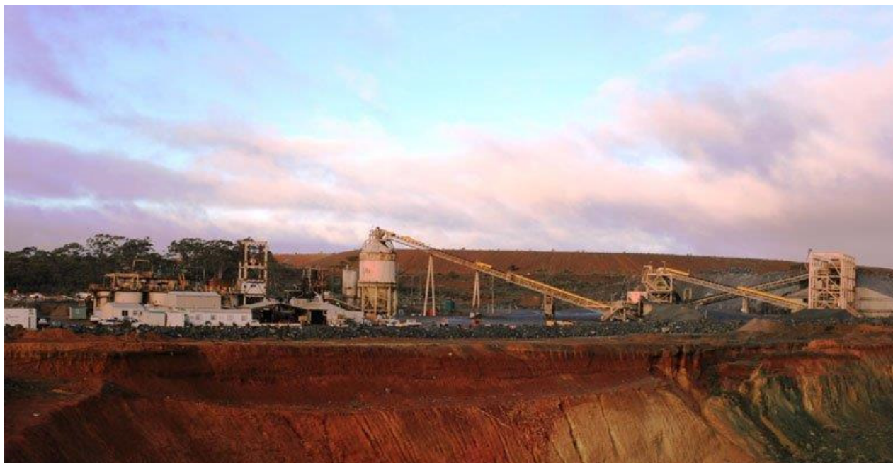
Greenfields Mill, Coolgardie Western Australia
