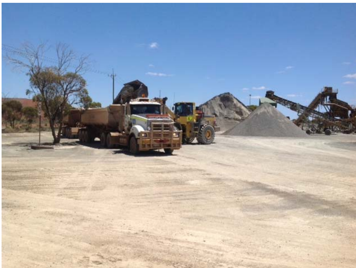
Figure 2 – Commencement of Crushing and Sampling - February 2016
