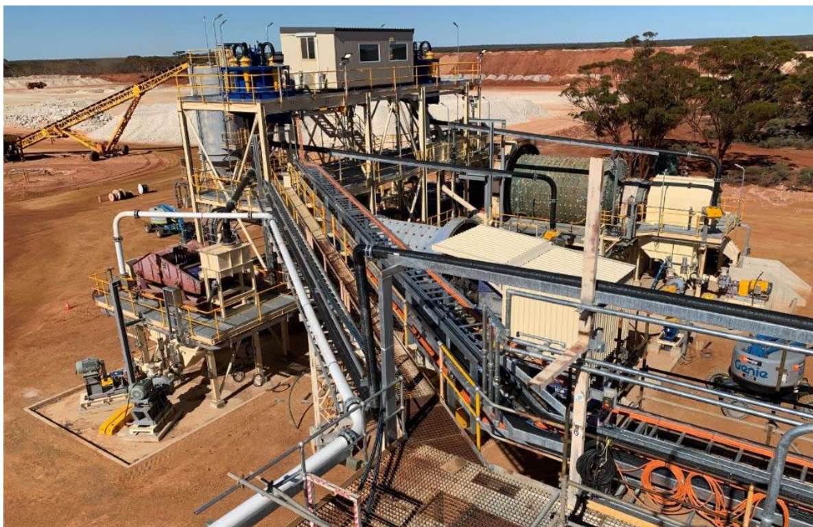
Jaurdi Gold Project – SAG Mill and Ball Mill Area, 28 May 2019
