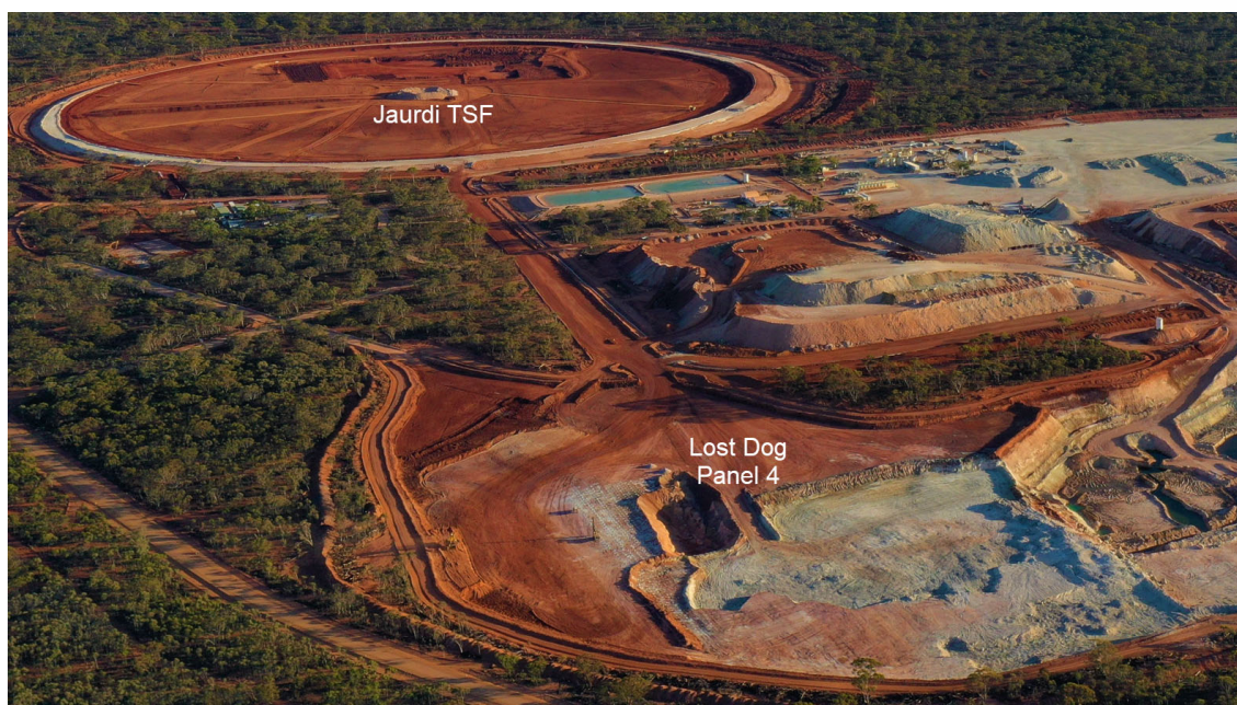
Jaurdi TSF – Earthworks 75% complete
