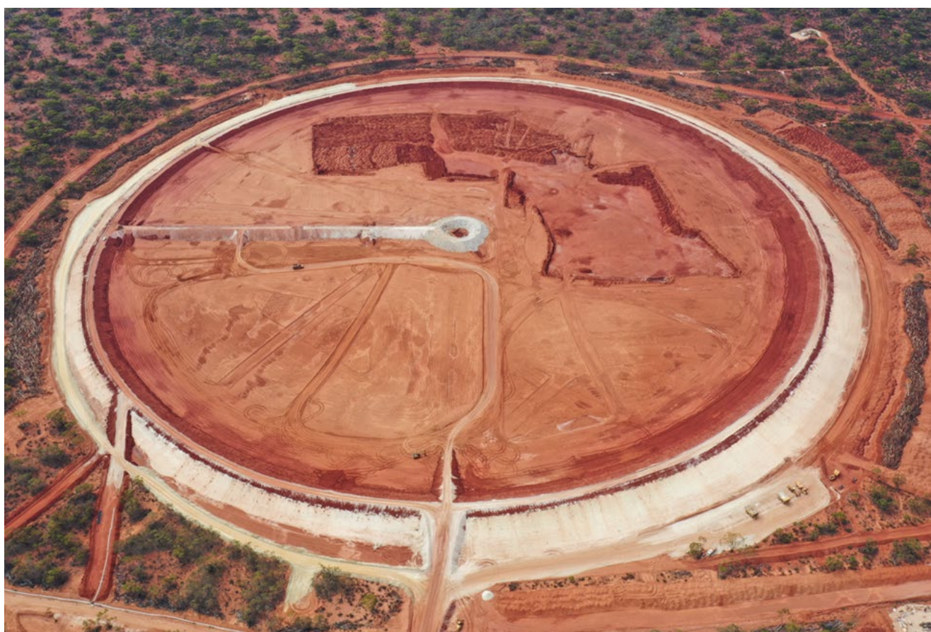
Figure 1: Jaurdi TSF earthworks
