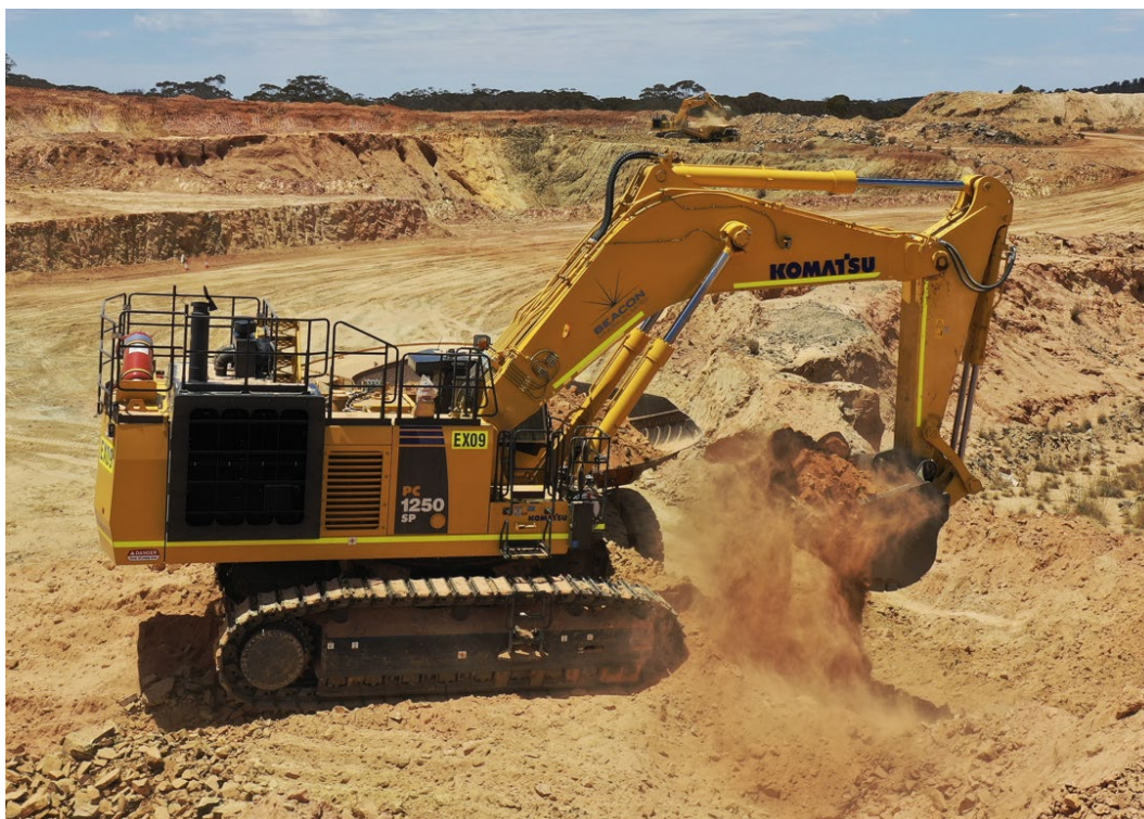
Figure 2 - Komatsu 1250 SP-8R Excavator at MacPhersons
