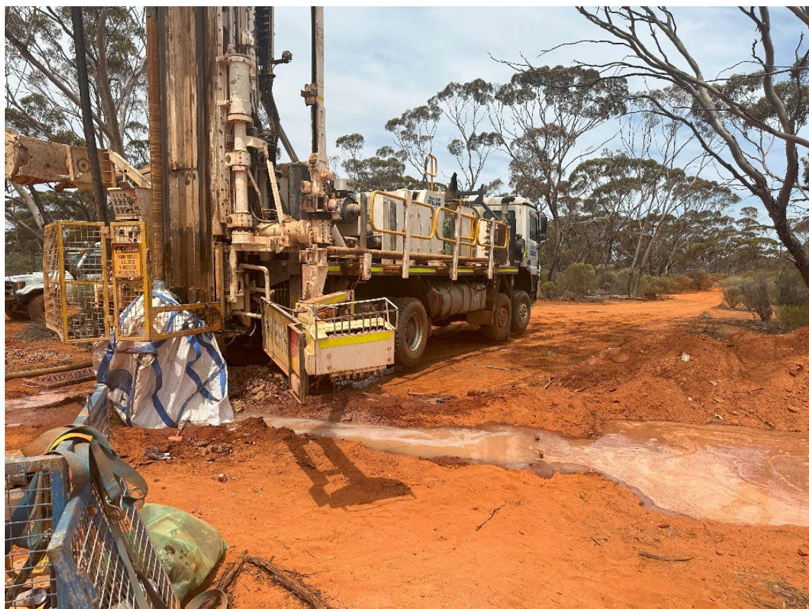
Figure 3: Water bore drilling east of Panel 3
