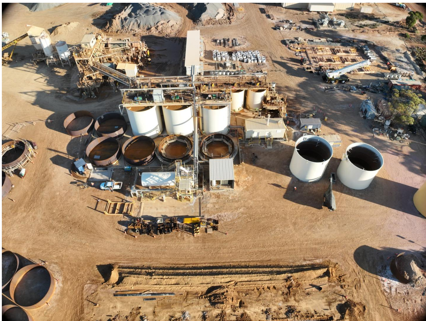
Image 3 – Jaurdi Gold Project Mill Upgrade – 28 April 2026
