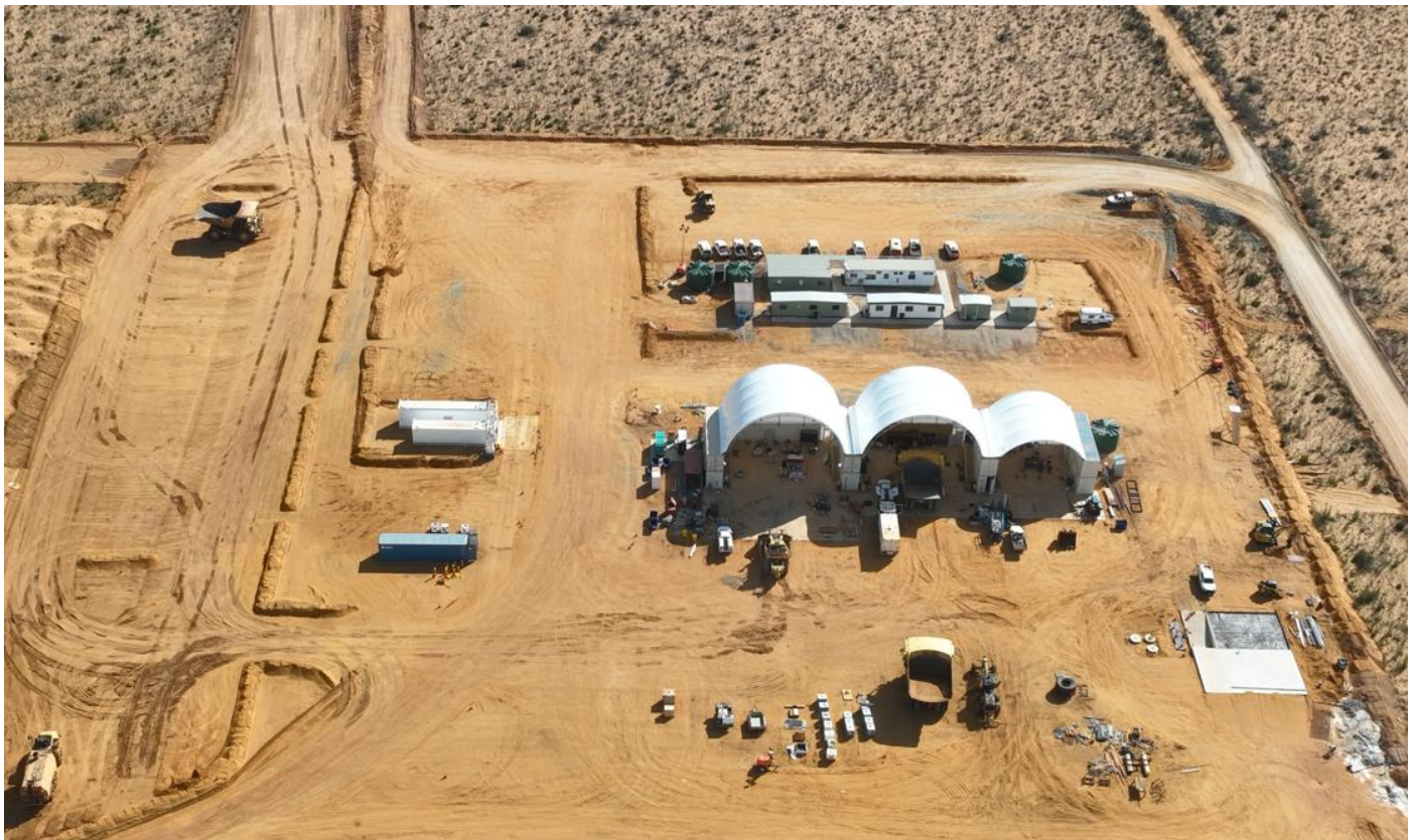
Image 2: Workshops and Infrastructure 20 April 2026
