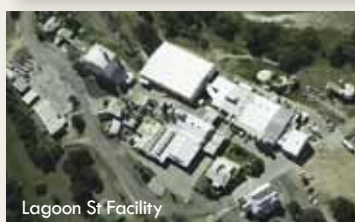
Bega Co-operative Creamery Company building
