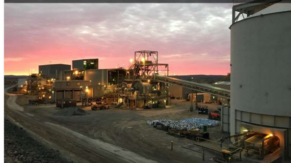
750,000tpa capacity processing facility
