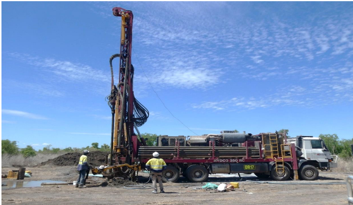
Figure 2: RC Drilling (Phase VI) at Sorby Hills.
