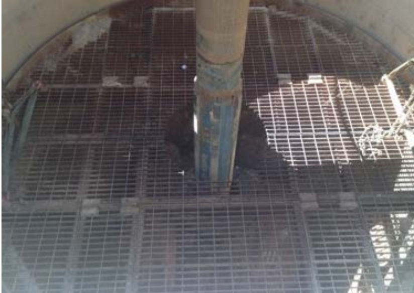
Figure 2: 3m diameter ventilation raisebore broken through to surface
