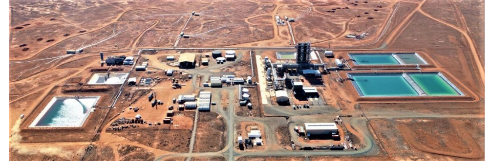
Honeymoon Processing Plant and Wellfields, South Australia
