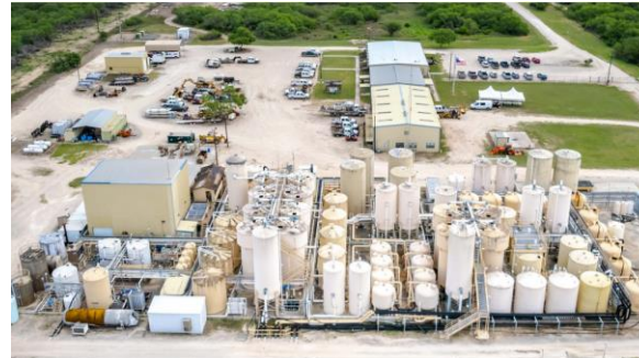
Alta Mesa Central Processing Plant, Texas, USA
