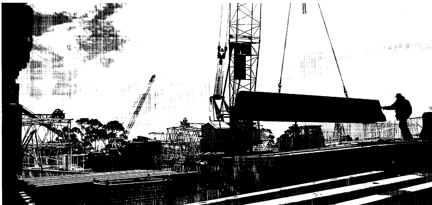
200 tonne pin jib crane.
