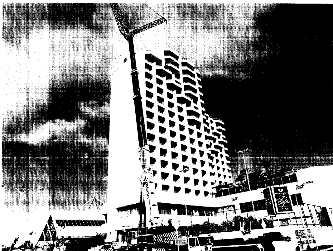
200 tonne all terrain crane.
