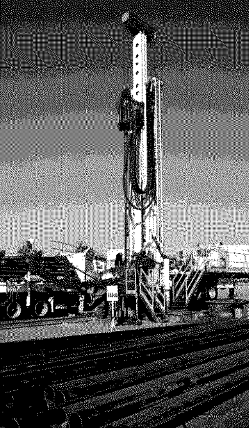
Tipton West Rig and Pipes
