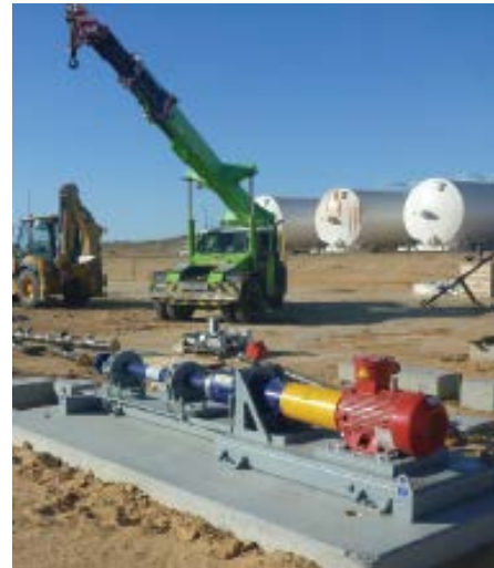
Construction of Pennington facility in ex PEL 91
