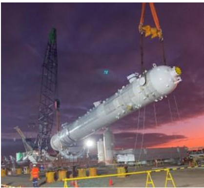
Waitsia Stage 2 CO 2 absorber lift
