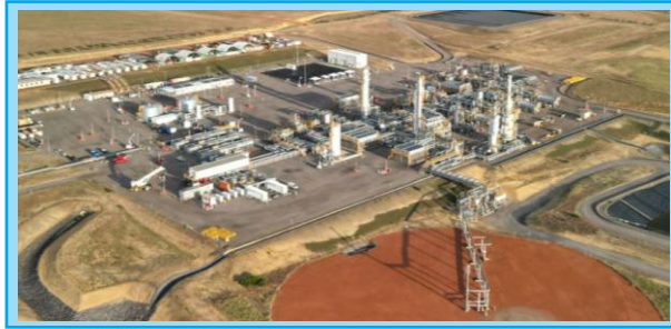
Waitsia Gas Plant
