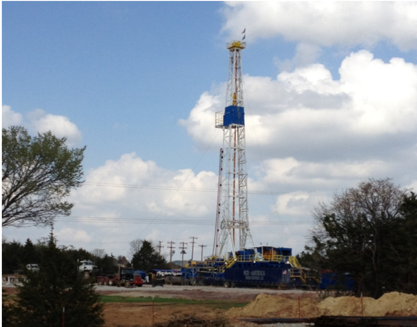
Jerry Scott Rig #5 Drilling, Noble County
