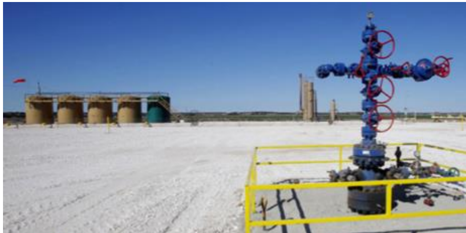
First cross-unit (long lateral) horizontal well drilled in Blaine County, Oklahoma Note: this is not an asset of Brookside Energy or Black Mesa
