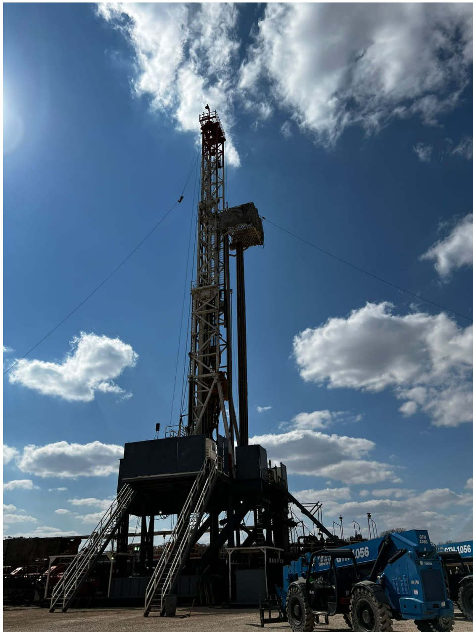
Figure 1. Kenai Rig 18 drilling the Flames Well
