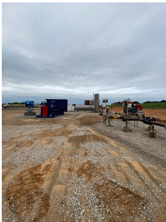
Figure 1. Plumbing in of surface production facilities
