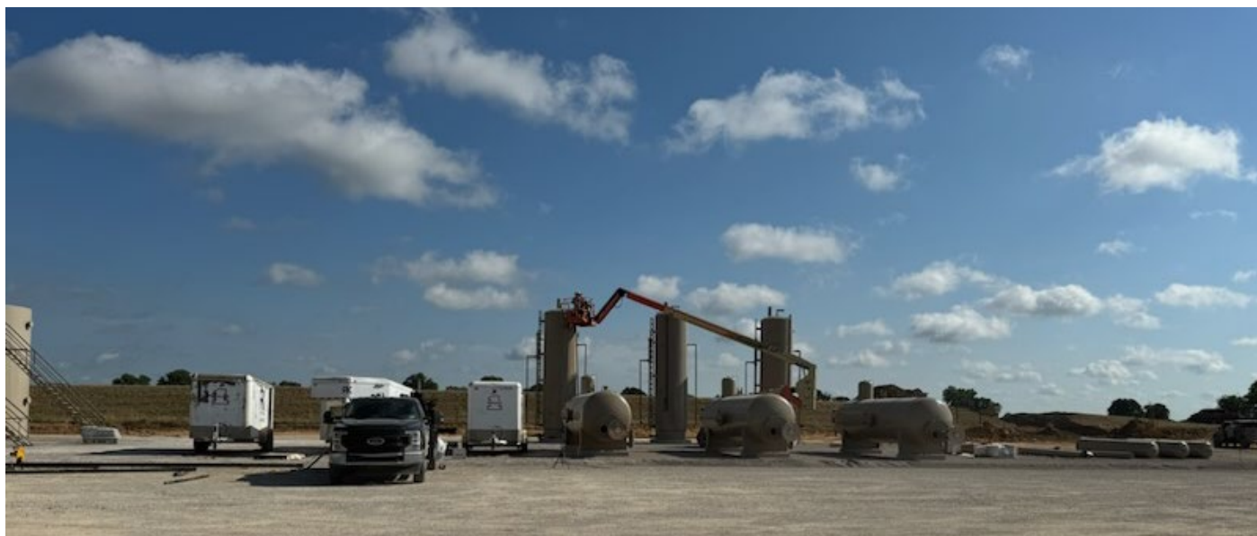
Figure 2: Setting of surface production equipment including the 18-tank battery on the Sanford Pad location.
