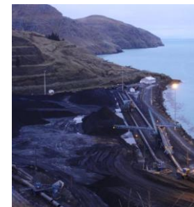
Coal stockpiles at the Port of Lyttelton
