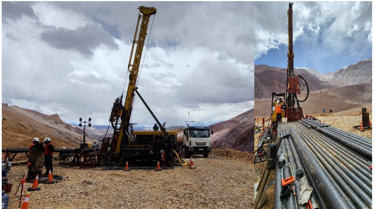
Figure 5: Drilling – Tambo South hole TMT-TSU-DDH-001.
