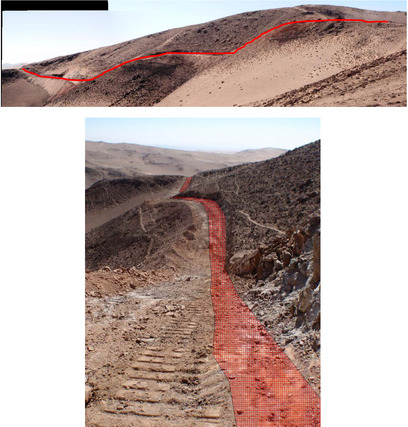
Figure 1 – Top, Long section view looking north west, of approximately 500m of strike length of the Panga vein which has had overburden removed – red line shows approximate position of the vein. Bottom – Looking south west along approximately 500m strike of the Panga vein showing over burden removed in preparation for bulk sampling – Red gridded area is mapped copper bearing vein.
