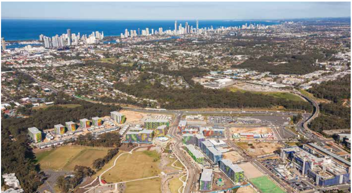
BSA | Build Parklands Project on the Gold Coast consisted of design and installation of Fire Detection, Fire Sprinklers, Fire Hydrants, Hose Reels, Fire Extinguishers and Occupant warning Systems to 18 midrise towers contained within 5 super lots. The site will contain 1,252 residences and 5 804m2 of retail space. In late 2017 Parklands Project will be transformed into the 2018 Commonwealth Games Village.
