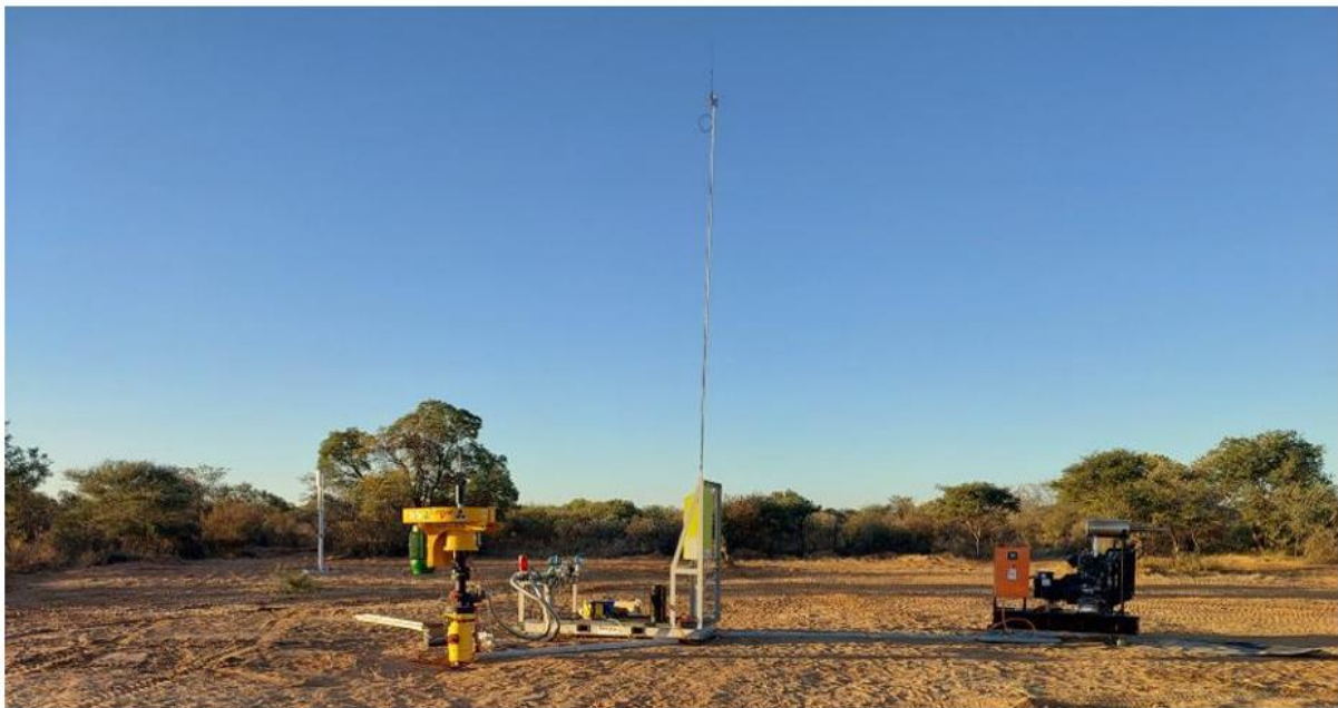
Figure 4. Serowe-3.4A Well and Surface Facilities (Source: Botala)
